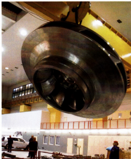
Assembly of the new runner for the pumped-storage hydroelectric power plant Dlouhý Stráně followed a 14-month-long manufacturing process.
